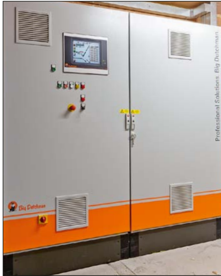
Control cabinet with amacs module »OptiSec manure drying tunnel«
