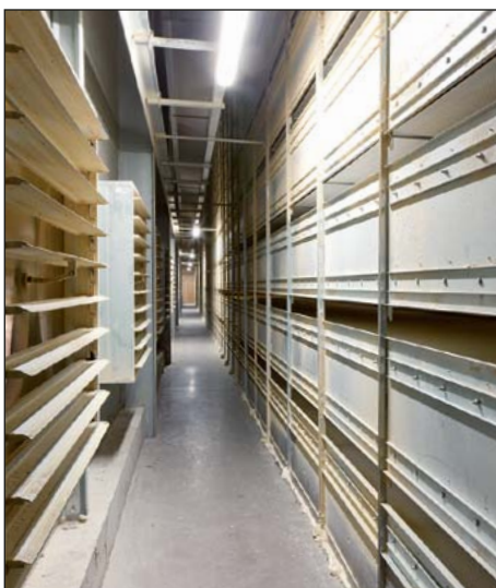
Pressure corridor with a positive pressure of approx. 25 Pa
