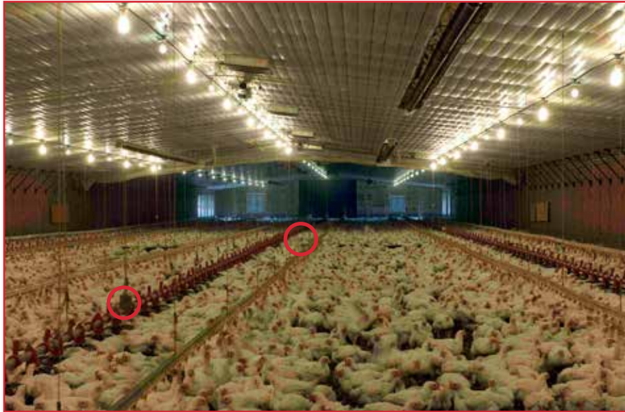
Figure 13: Correct location for temperature and humidity sensors.
