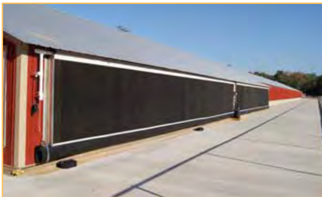
Figure 113: Example of a cooling pad.
