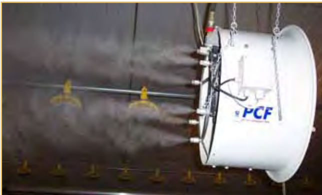
Figure 112: Example of spray cooling system.
