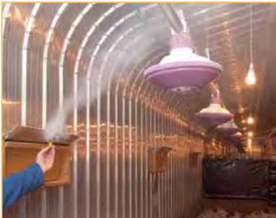
Figure 106: A direction plate fitted to an air inlet.
