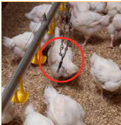
Figure 16: Correct location for temperature/humidity sensors.
