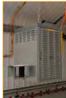
Figure 100: Examples of different house heating systems (from left to right, canopy brooder, whole-house heating, and space heater).
