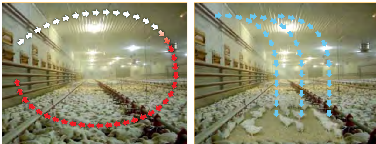
Figure 107: Illustration of airflow into the house. The picture on left shows a correct fast airflow during minimum ventilation, the picture on right shows an incorrect slow airflow during minimum ventilation.
