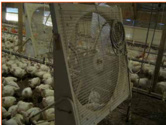
Figure 29: Circulation fans in a naturally ventilated house.
