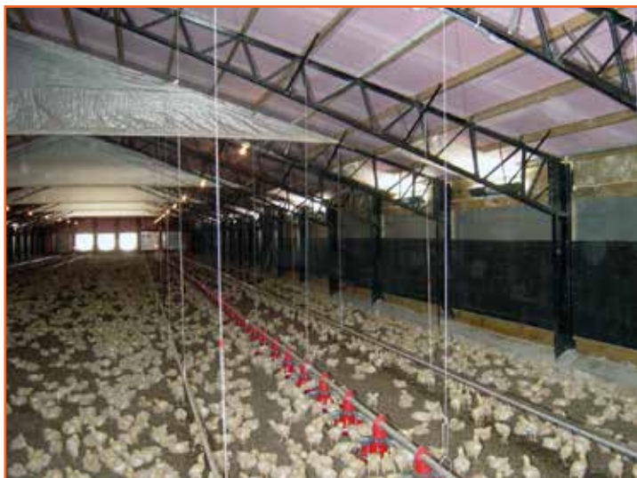
Figure 37: Internal view of house in transitional ventilation mode. Inlets are fully opened and the tunnel fans are running. Bird distribution shows birds are comfortable.
