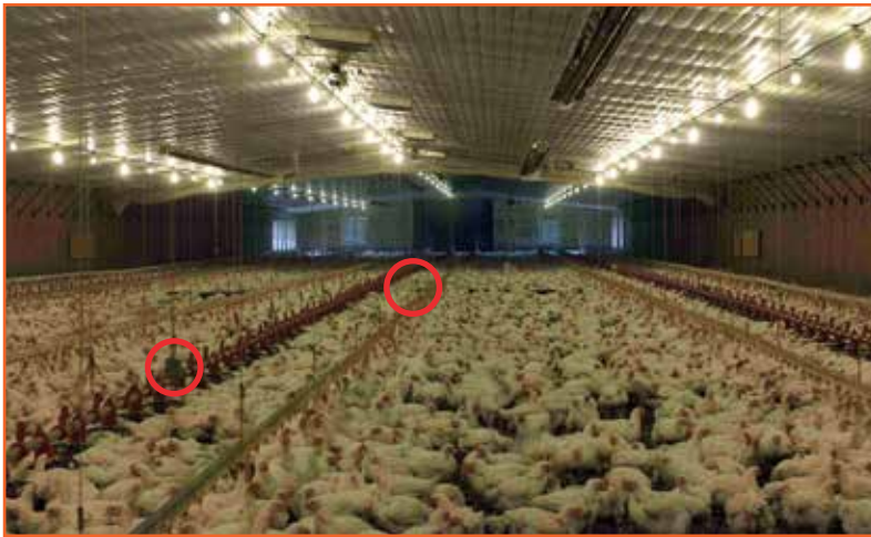
Figure 13: Correct location for temperature and humidity sensors.
