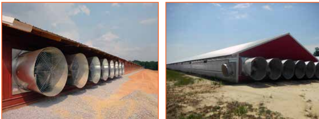
Figure 40: Example of a typical tunnel ventilated house.
