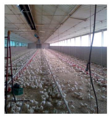
Radiant system "**INFRA BAF DES**" heats through radiation and convection with destratification effect, directing heat only to specific areas
